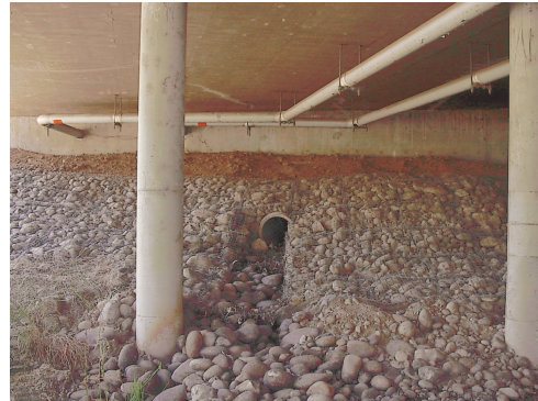
INTERSTATE I-80 UNDERPASS (BARRIER #2 ON GIS MAP)
