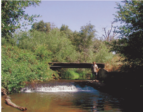
CONCRETE DAM AT CONFLUENCE (BARRIER #1 ON GIS MAP)
