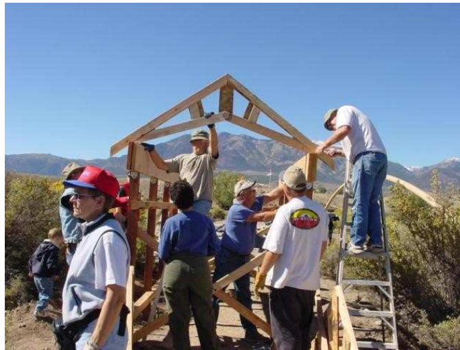
Marysvale Kiosk construction. Photo courtesy of Max Reid.
