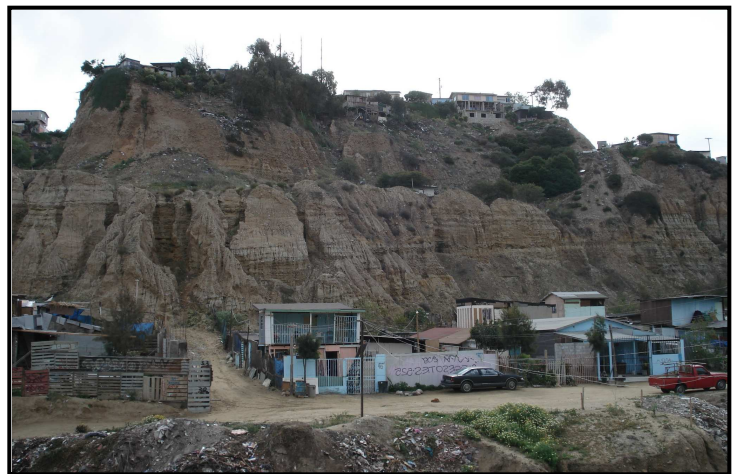
Figure 15. Erosion of canyon walls. (Source: R. Keane-Dengel, May 2007).
