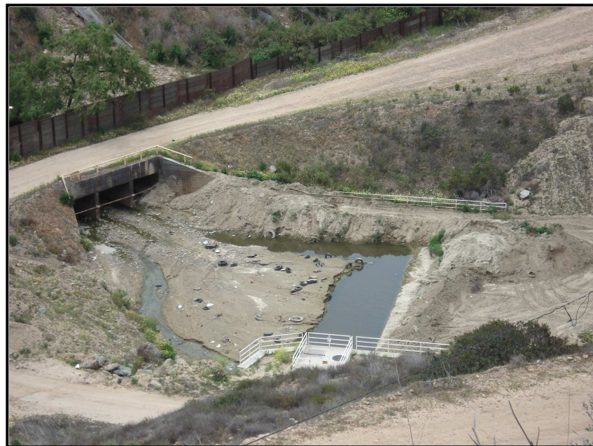
Figure 18. Sediment settling pond on the U.S. side of the border (Source: R. Keane-Dengel, May 2007).
