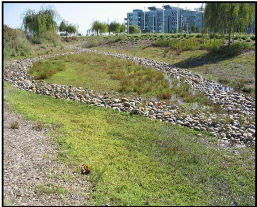
Figure 35. Photo of dry detention basin (Bill Southard, DES Architects)
