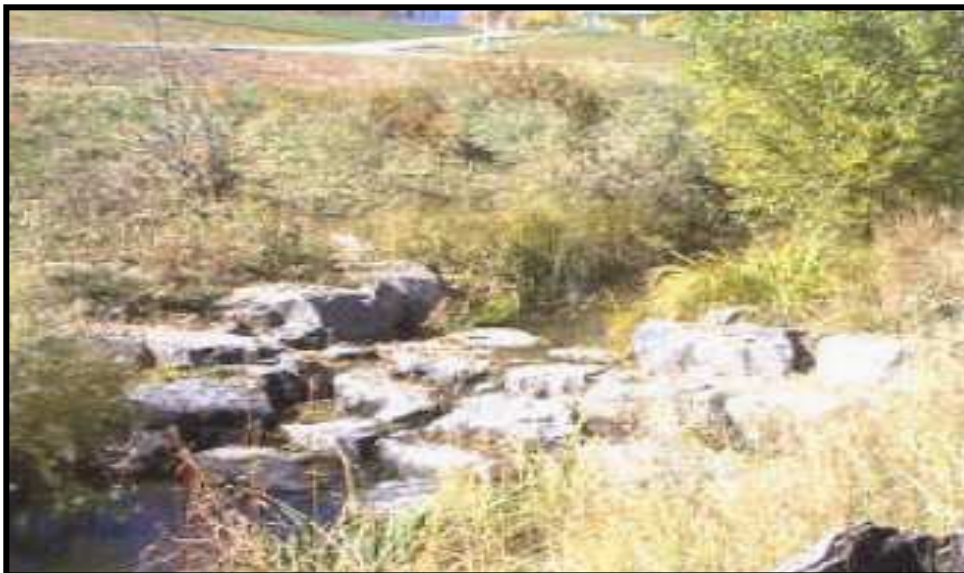
Figure 44. Channel grade control with riprap (Urbonas, 2003).
