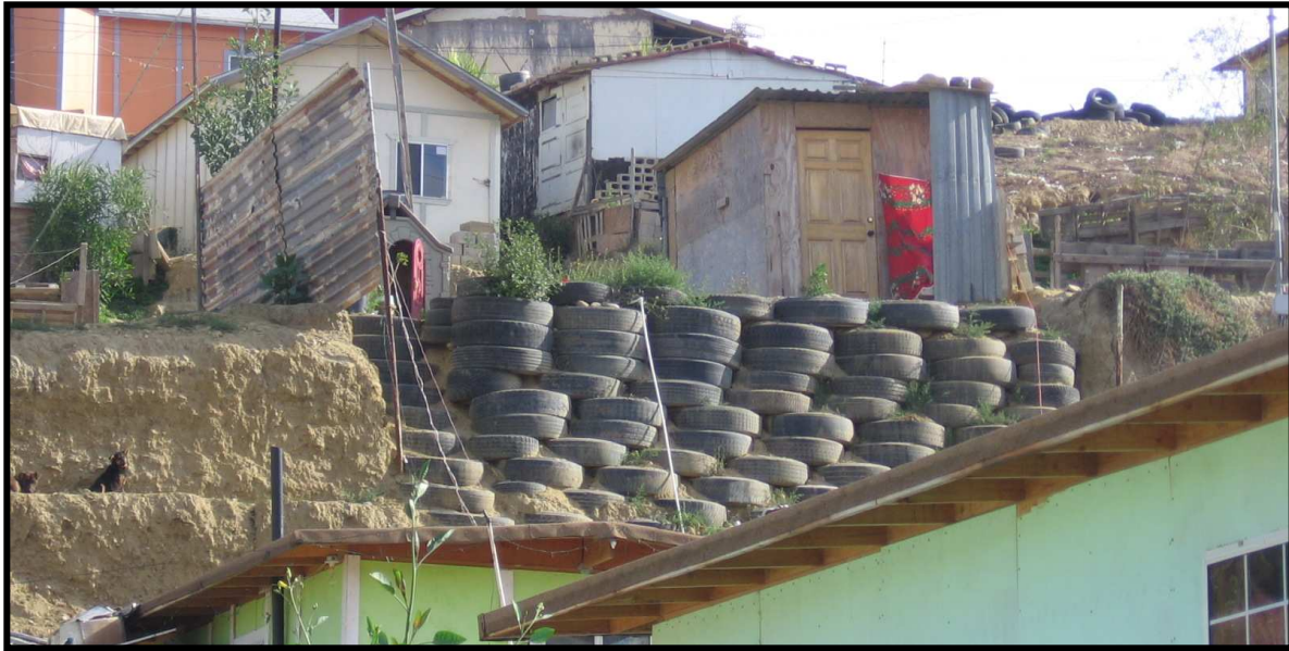
Figure 46. Unreinforced tire retaining wall in Los Laureles Canyon. (Source: N. Virgilio, 2007.)
