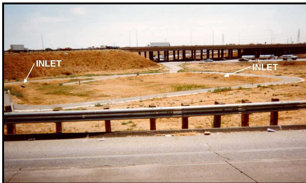
Figure 32. Typical infiltration basin (California Stormwater Quality Association, 2003).
