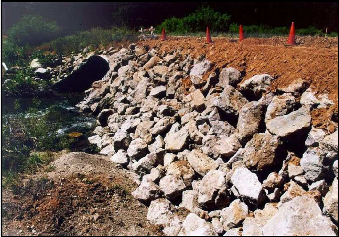
Figure 45. Riprap used for channel protection ( http://www.fs.fed.us )
