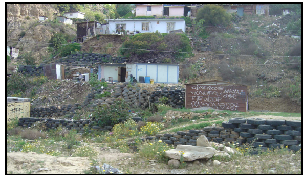
Figure 7. Tire retaining wall structures
