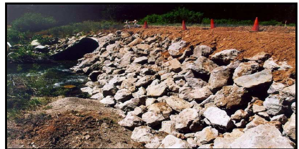
Figure 8. Riprap channel stabilization
