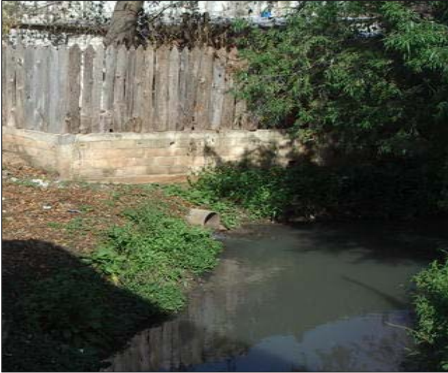
Picture 5.1. A sewage outfall into the Río Amarillo at a location on the northern end of the urban center of the watershed.
