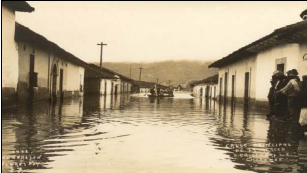
Picture 3.3. Flooding in San Cristóbal, circa 1932 (García García 2005).
