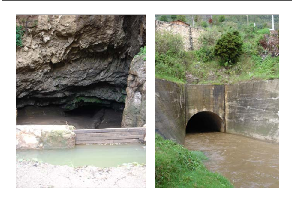
Picture 3.1. The image on the left is the natural outlet of the watershed as it looks today. This outlet has been blocked off and the river diverted from its natural path to the constructed tunnel about 25 meters away. Water now drains directly to the tunnel, shown in the image on the right.
