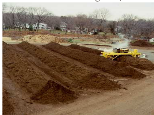
Figure 7-2: Open air windrow piles
