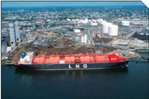
Figure 1 - Onshore Facility. Source: Spec Engineering
