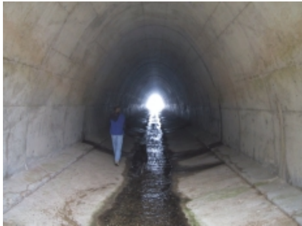
The interior of the culvert passing beneath Highway 101 at Arroyo Hondo.
