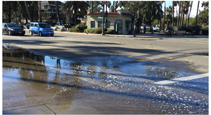
Above: Cabrillo Boulevard flooding. Photo Credit: Laura Nicholson
