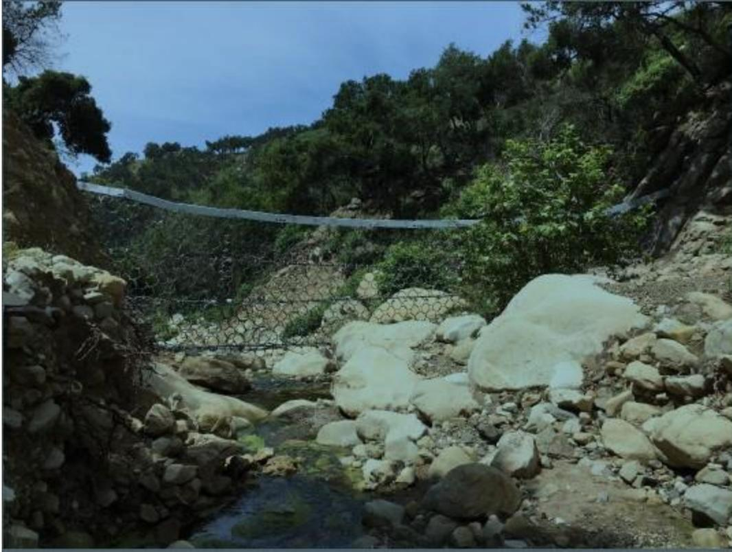
**Figure 3.34** - Ringnets on Cold Springs Creek. Source: (SCHR)
