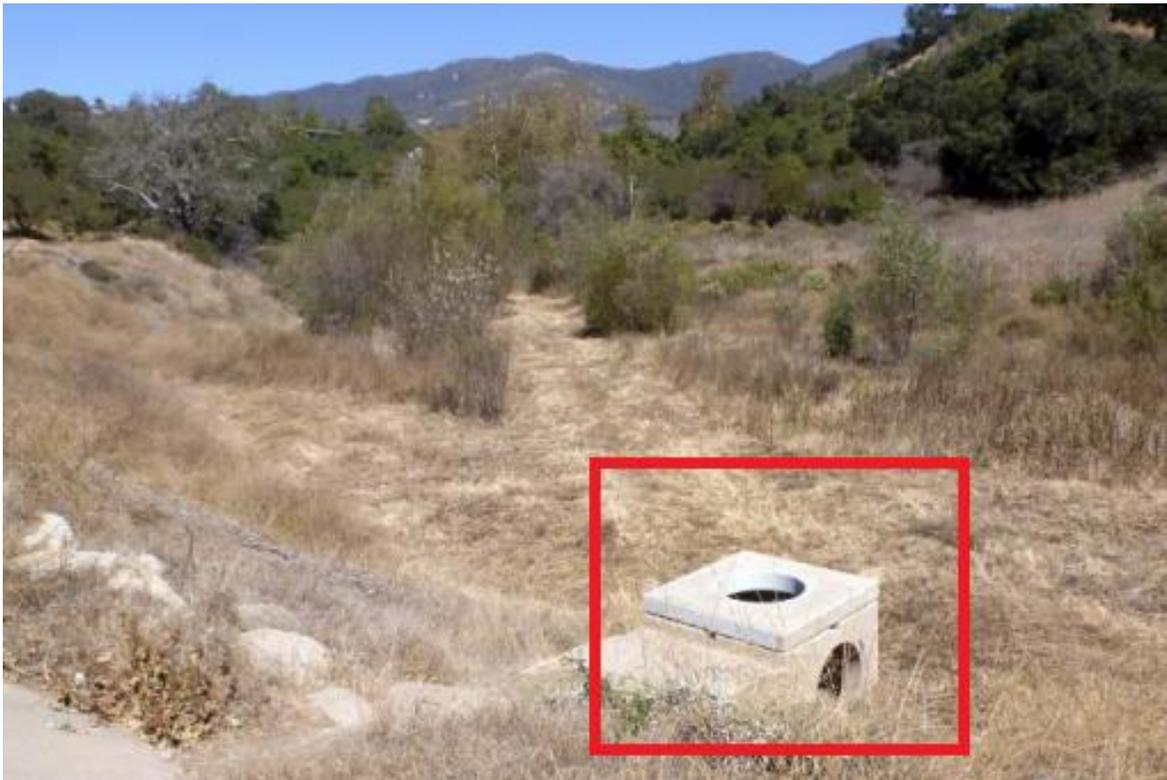
**Figure 3.37** - Example of boxed outfall from San Antonio Debris Basin. Source: (SBCFCD)
