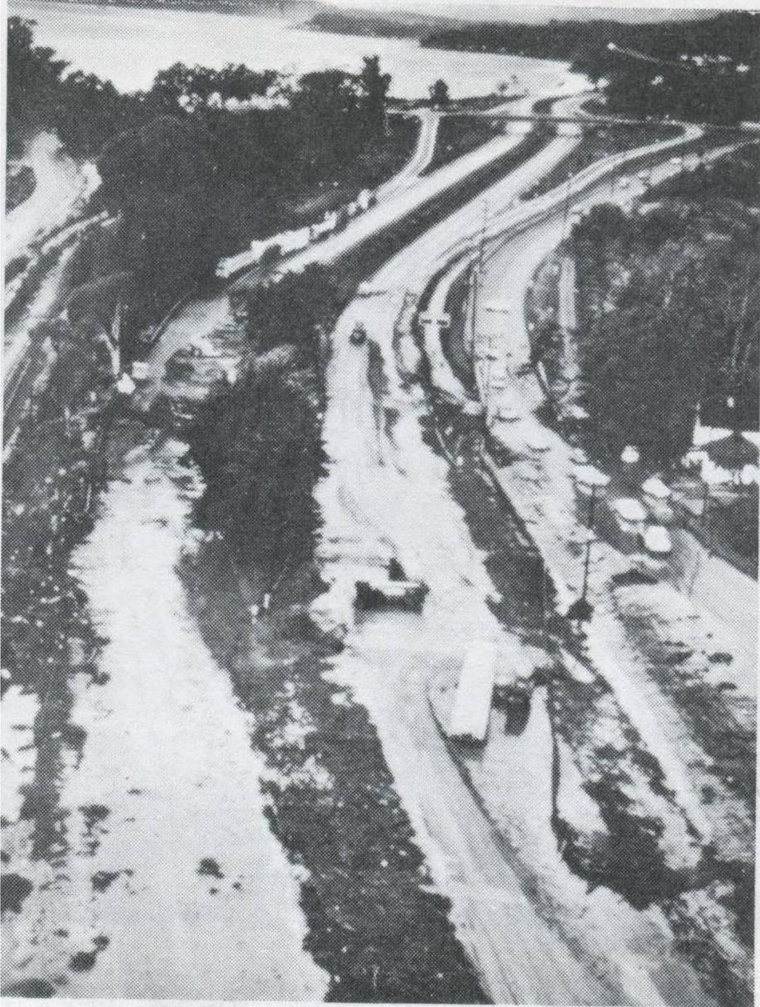
**Figure 3.10** - View of U.S. 101 overtopped with mud after a debris flow post-Romero Fire. Source: (SB Bucket Brigade)
