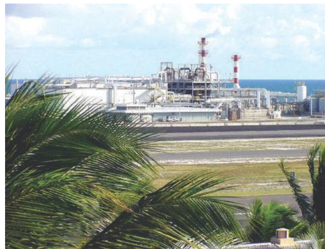
Johnston Atoll Chemical Agent Disposal System (JACADS) building, Photo: U.S. Army Chemical Materials Agency.
