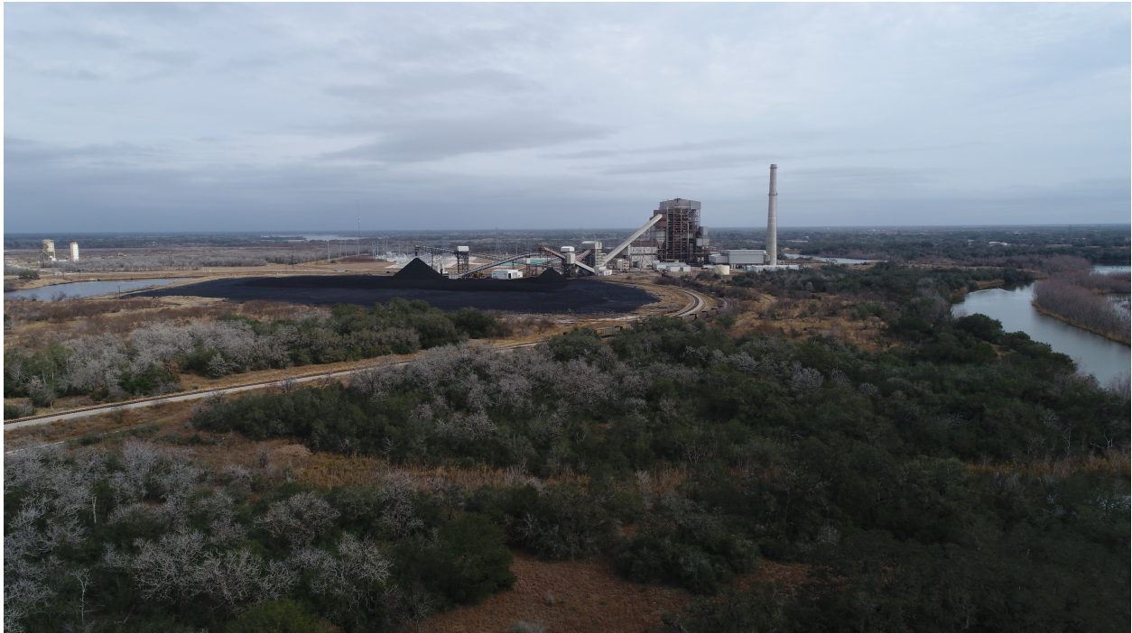
Figure 11: Coletto Creek Power Plant.
