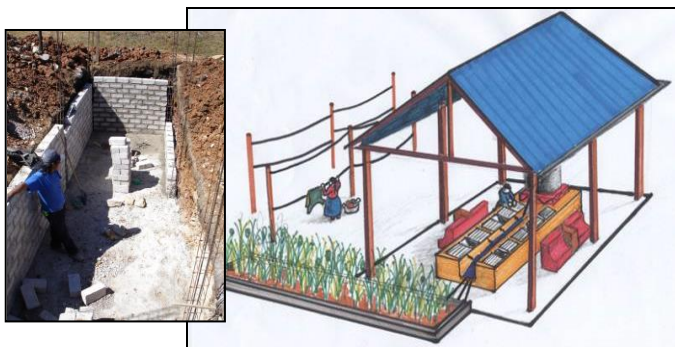
Figure 8. Construction in progress and a conceptual drawing of the finished EcoLavadero
