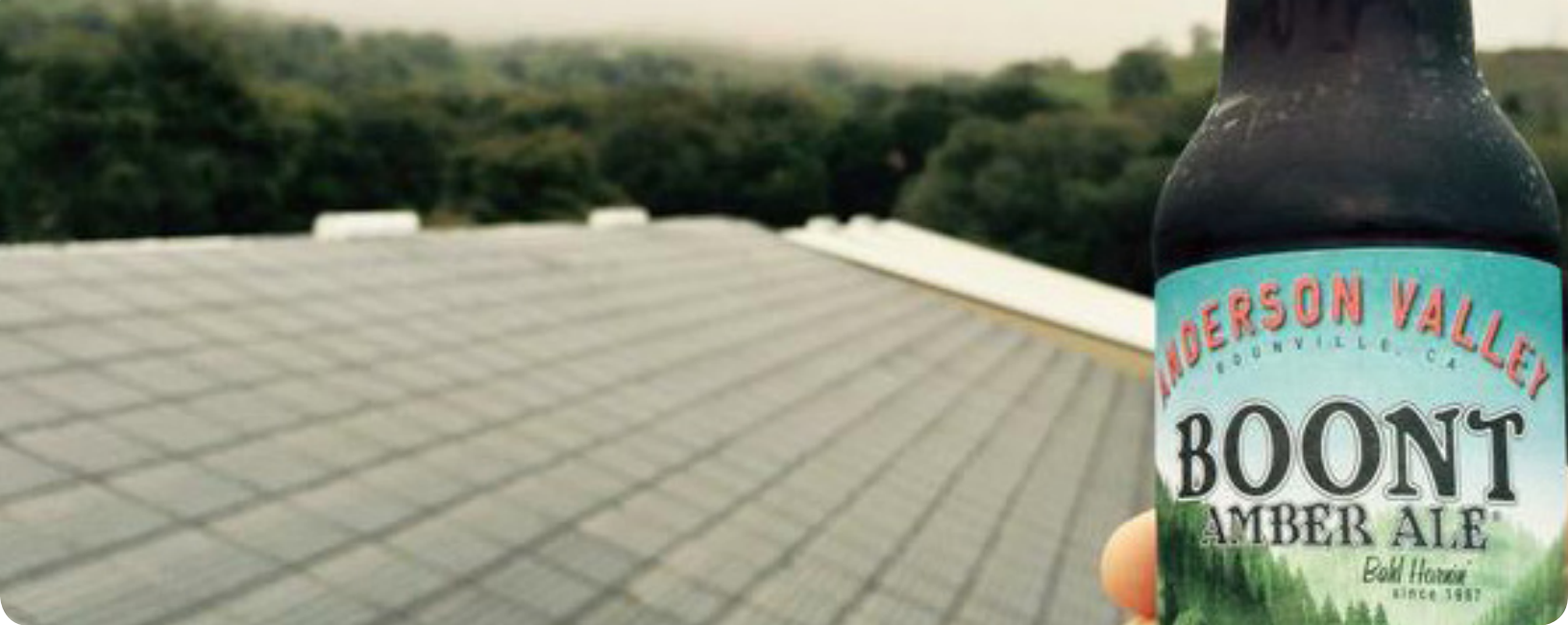
Anderson Valley solar installations. Source: Anderson Valley
