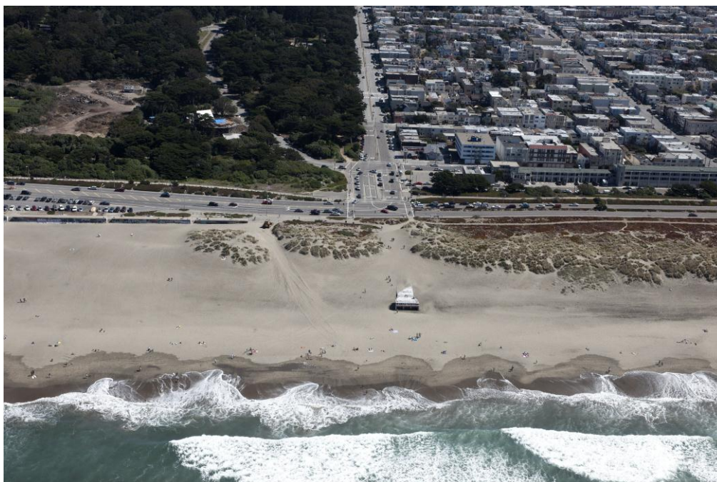
Figure 9: Outfall structure located along Ocean Beach.
