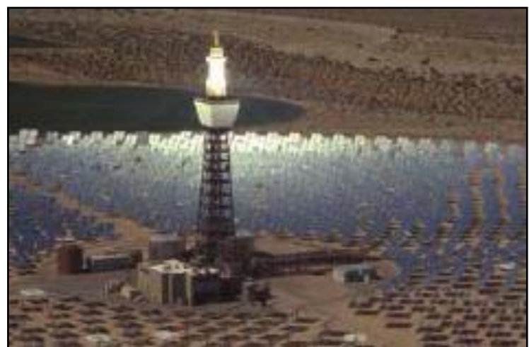
Figure 2. An example of power tower technology. This is a 10 MW capacity pilot project in Barstow, CA. (Source: DOE)
