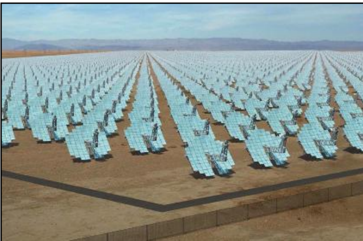
Figure 3. The 750 MW Imperial Valley Solar Energy Project is an example of Parabolic Dish/Heat engine technology. (Source: CEC)
