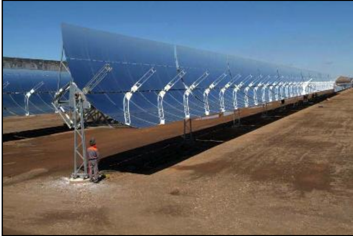
Figure 1. The Blythe Solar Power project is an example of a Concentrating Solar Thermal (CSP) Parabolic Trough. (Source: CEC)
