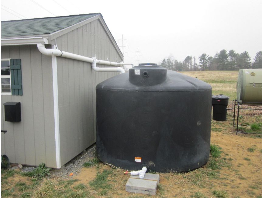
Figure 4. Large rain cistern. Cisterns used in the Waller-3 Rain Catcher Pilot project are able to hold 1,000 gallons of captured rainwater. Source: gardening.stackexchange.com .
