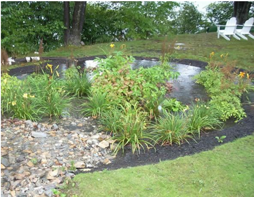
Figure 5. Rain garden. Rain gardens in the Waller-3 Rain Catcher Pilot Project are approximately 100 cubic feet. Source: U.S. Environmental Protection Agency.
