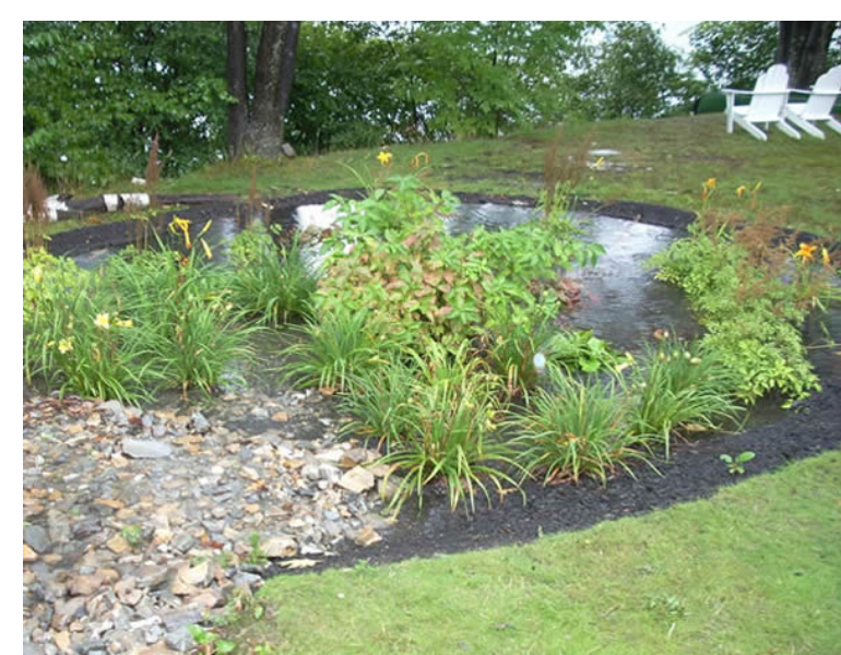
Figure 3. Rain garden. Rain gardens in the Waller-3 RCPP are approximately 100 cubic feet. Source: U.S. Environmental Protection Agency.
