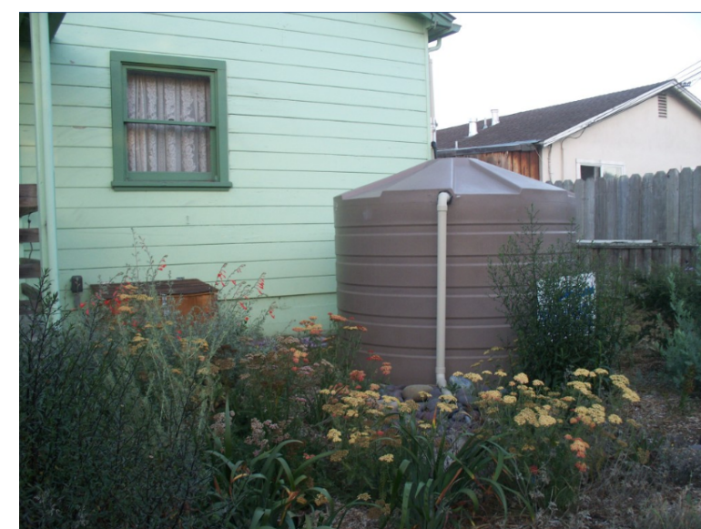
Figure 2. Large rain cistern. Cisterns used in the Waller-3 RCPP are able to hold 1,000 gallons of captured rainwater. Source: gardening.stackexchange.com.
