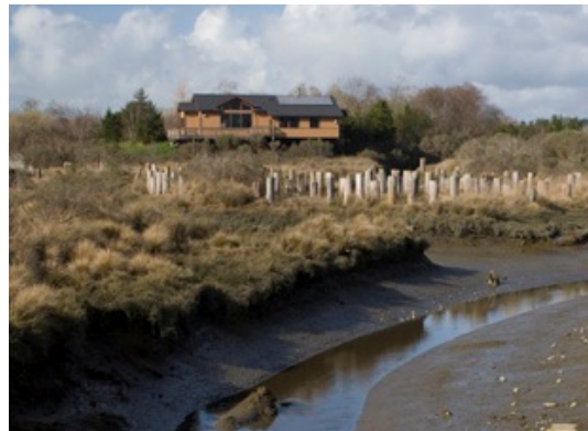
Figure 9. Arcata Marsh Interpretive Center (Source: Arcata's Wastewater Treatment Plant and Arcata Marsh and Wildlife Sanctuary, 2009b)
