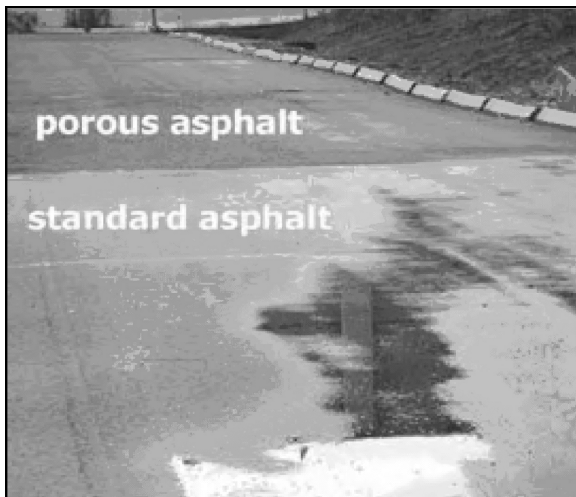
Figure W2: Comparison of Permeable Versus Standard Asphalt. [Courtesy of Truckee Meadows Regional Stormwater Quality Management Program and Kennedy/Jenks Consultants]
