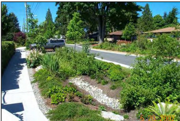
Figure W3: Photo of Biofiltration System in Seattle, WA [Courtesy of Truckee Meadows Regional Stormwater Quality Management Program and Kennedy/Jenks Consultants]
