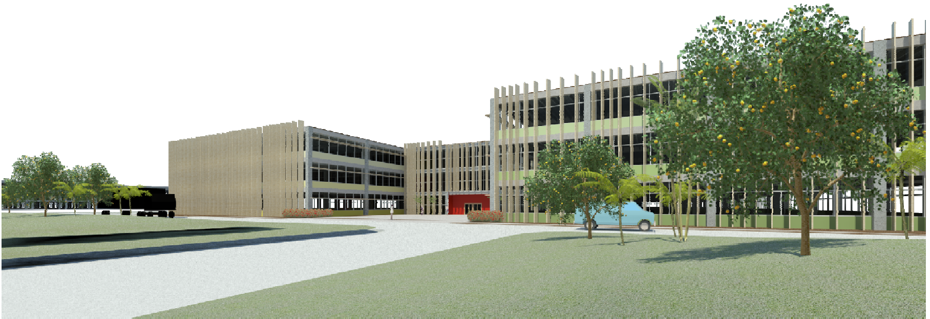
Front View of the Facility, Highlighting the Vertical Shading and Light Shelves
