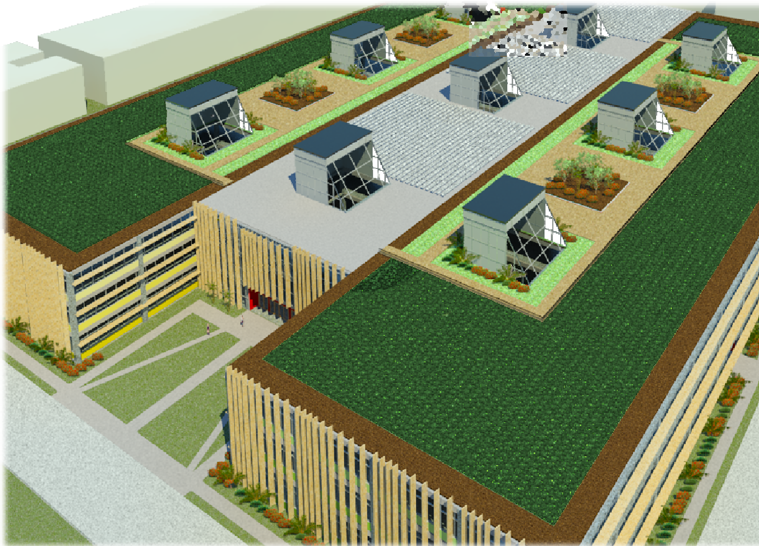
Overhead View of the Facility with Solar Chimneys
