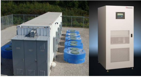
Figure 2.11 - Flywheel Applications: Right, 1-MW/15-min Beacon Power flywheel in an ISO ancillary service application, Left: Pentadyne GTX flywheel (Source: EPRI, 2010)
