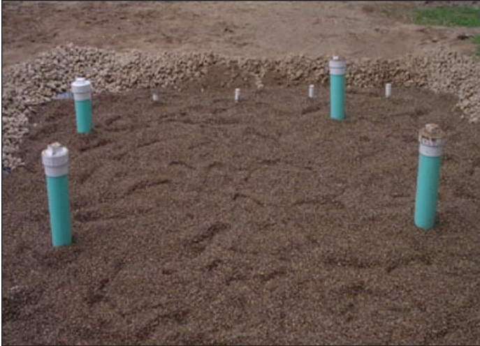
Figure 9. Pea gravel covering pressure laterals.
