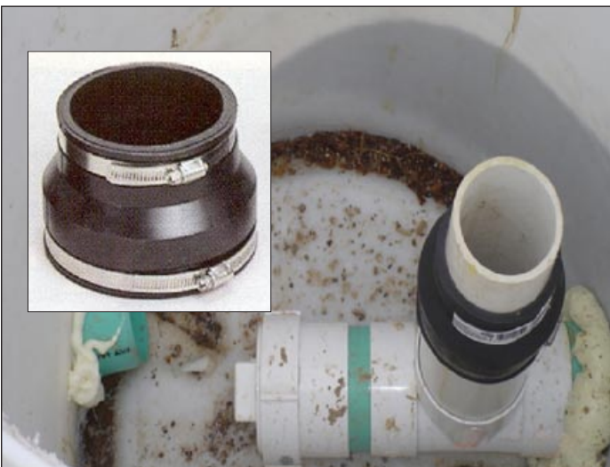
Figure 6c. Wetland water level adjustment showing the PVC to PVC 4" x 3" flexible sewer couple reducer.
