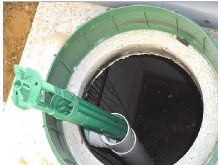
Figure 13. To clean a septic tank effluent filter, simply lift it out of the tank and hose it off. Let solids fall back into the tank.
