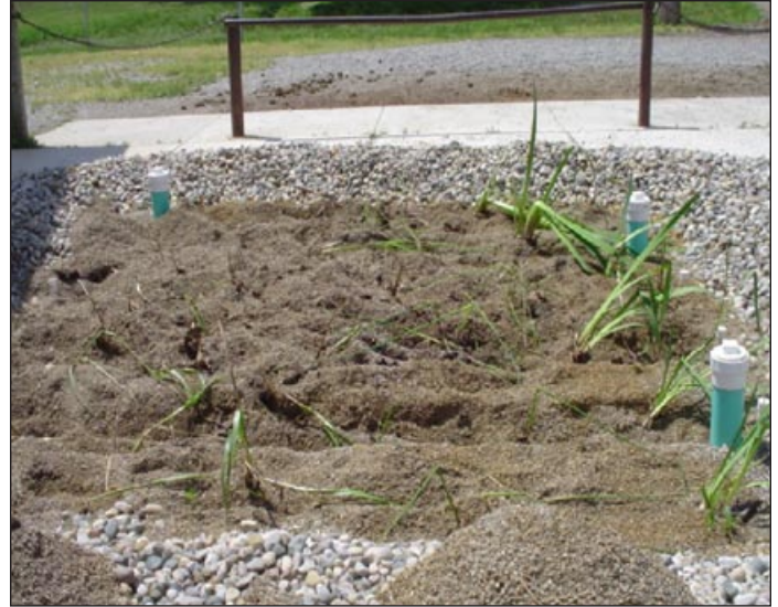
Figure 11a. Wetland immediately after planting.
