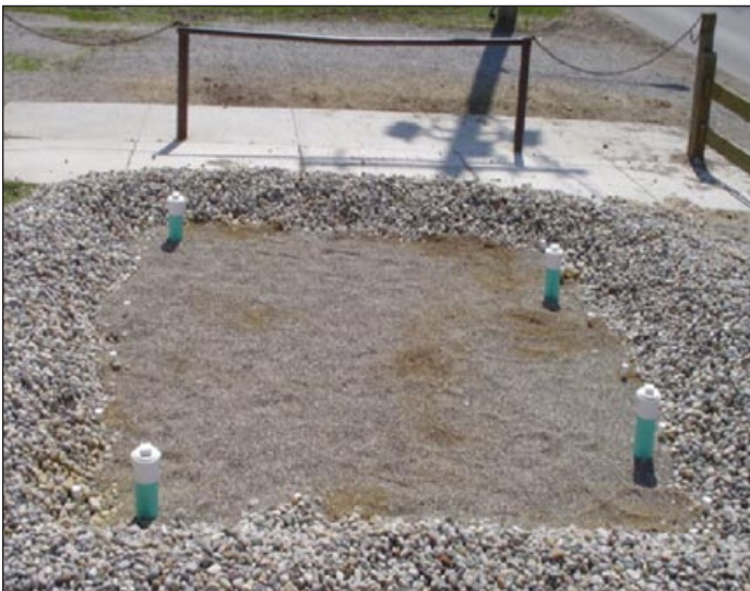
Figure 10. Finished RVF wetland with regular stone around edges.
