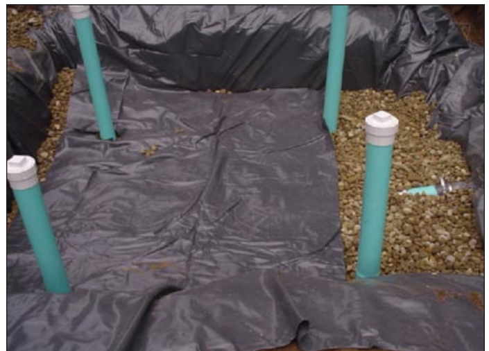
Figure 5. Upper or second liner covering 75% wetland cell.
