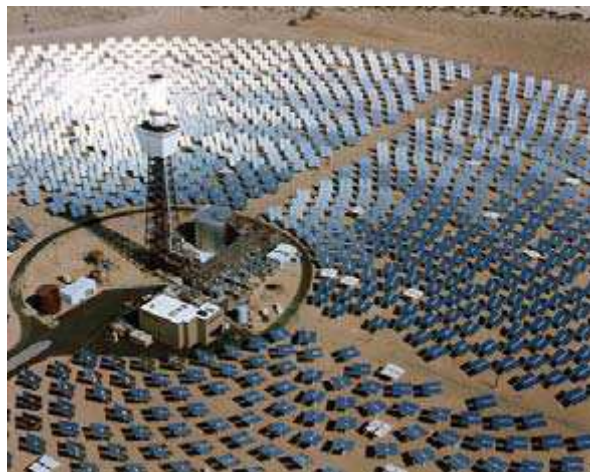
Figure 35. 10 MW Solar Two power tower system (NREL, 2006).
