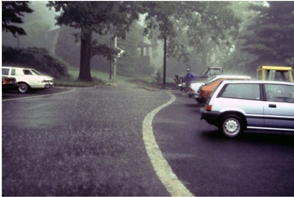
Figure 25: A photo of parking spaces during a heavy Pennsylvania rainstorm. The road to the left of the yellow line is paved with conventional asphalt, while the parking spaces to the right are porous asphalt.
