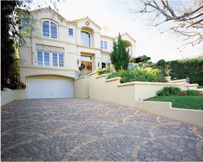
Figure 24: Decorative use of an interlocking paver system for a residential driveway (Barazani Pavestone)
