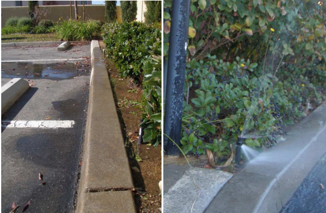
Figure 12 Examples of runoff from pooling and lack of mulch (left) and broken spray heads (right)
