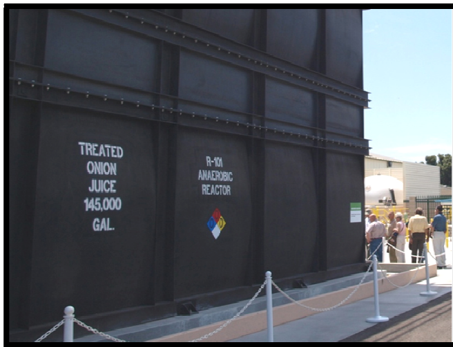
Figure 3 Gills Onions' 145,000 gallon anaerobic digester
