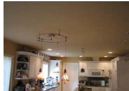
Image 5: Lights in ceiling add to air infiltration
