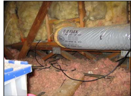
Image 2: Poor knee-wall air sealing.
