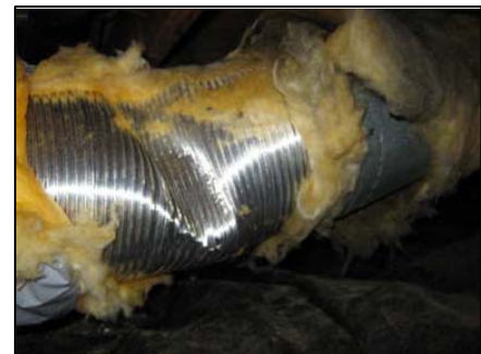
Image 4: Aluma-Flex is susceptible to damage.
