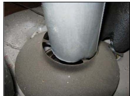
Image 3: Miss-match of vent pipe against draft-diverter.
