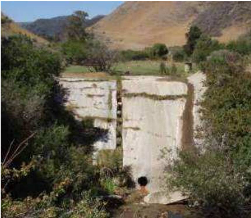
Figure 11: Santa Anita Dam located 1 km upstream from the ocean
