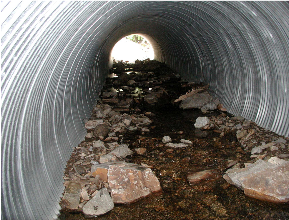
Figure 32: Example of an embedded culvert
