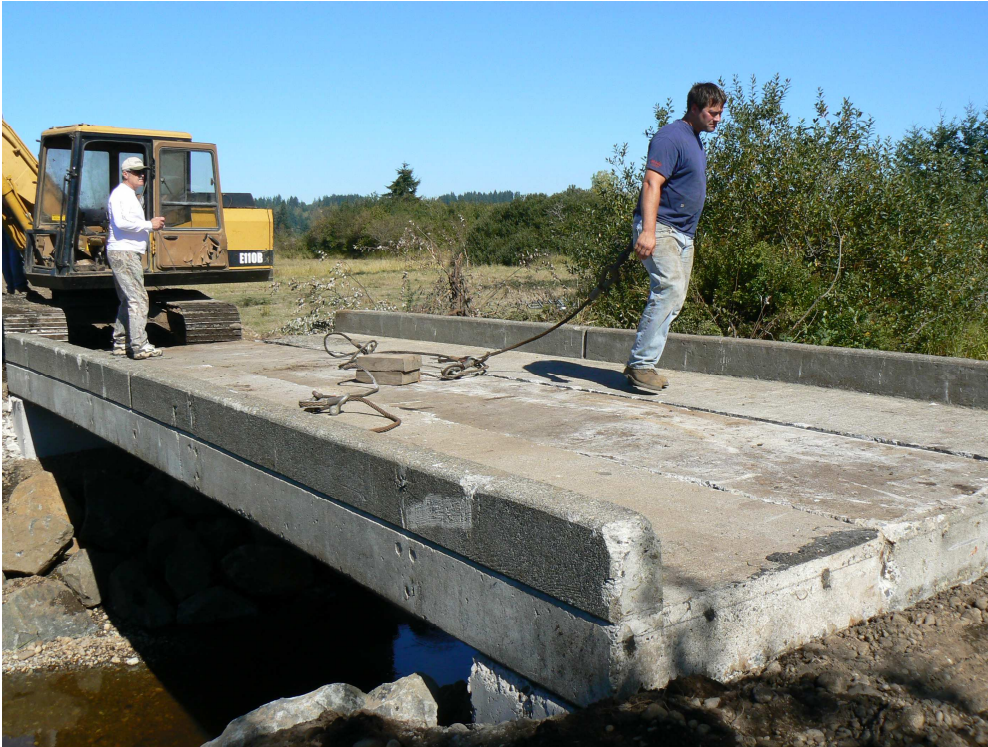
Figure 31: Precast Bridge Stream Crossing
