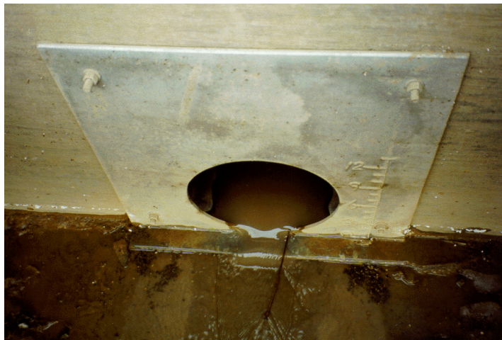
Figure 3.1 Orifice Plate at the Forebay Inlet
