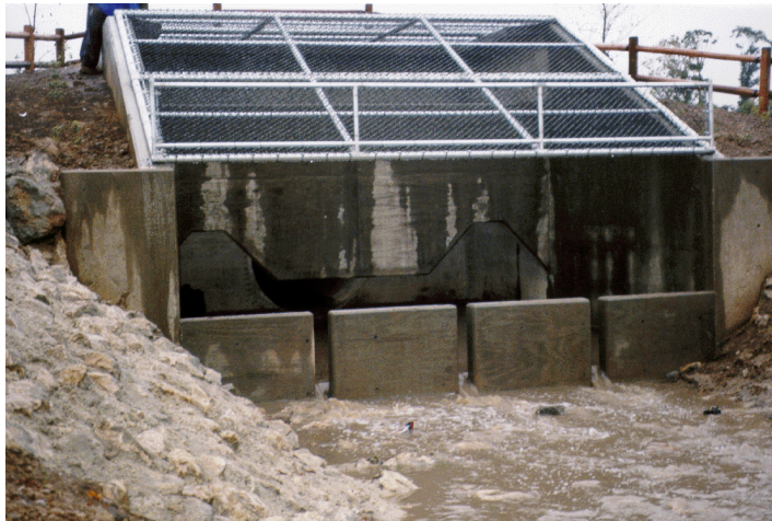
Figure 3.3 Energy Dissipator Discharge to the Natural Area
