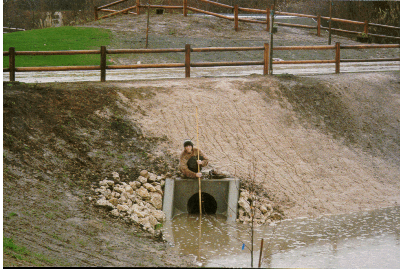
Figure 5.2 Erosion of Bioswale Banks
