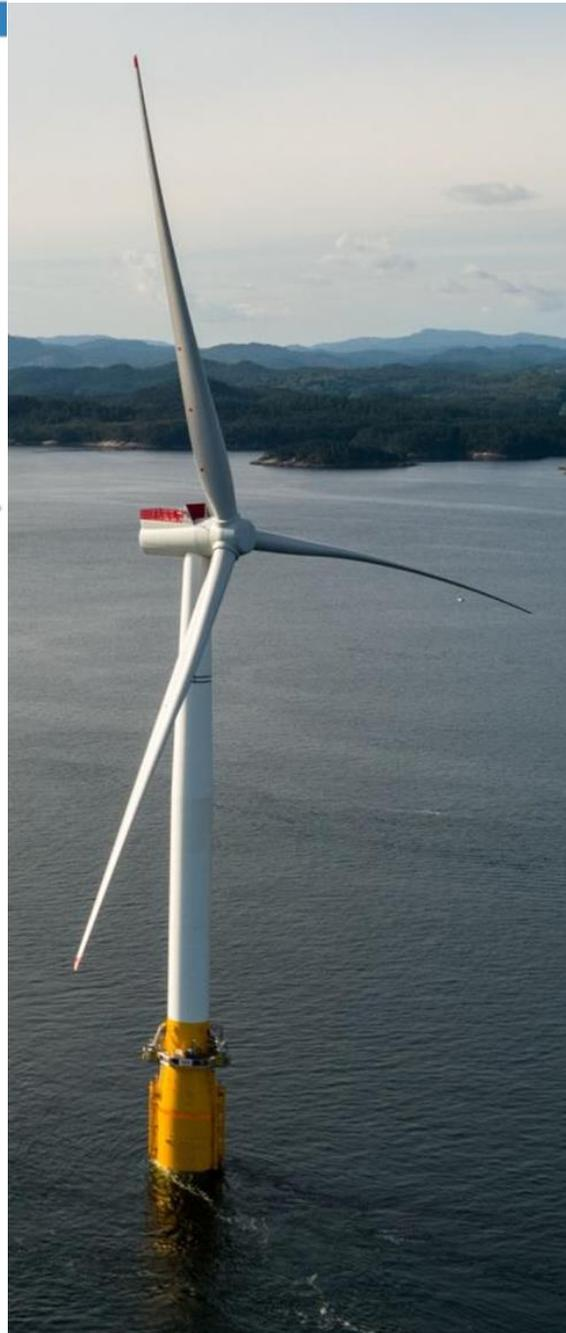
Figure 9. Original design of representative wind turbine, substructure, and mooring/anchoring system adapted from the Hywind Scotland commercial pilot park to deployment in federal waters off CA.<sup>40</sup>
